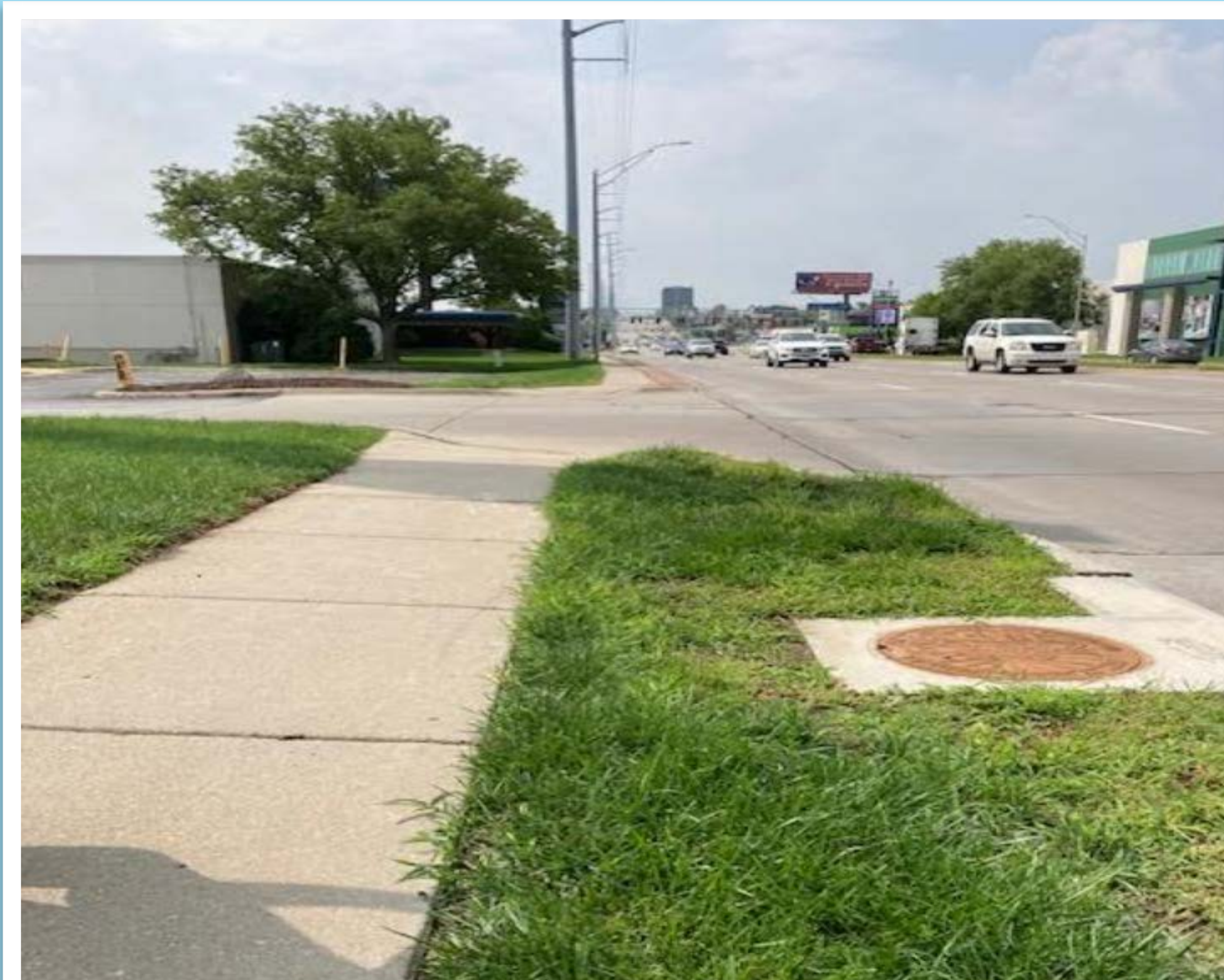
East side of 72nd just south of 72nd & Jones (adjacent to the parking lot for Michael's & Petsmart - facing south.) Notice the next section of sidewalk in the background of the photo has a reduced buffer of colored pavement vs. the wider buffer of vegetation in the foreground.
