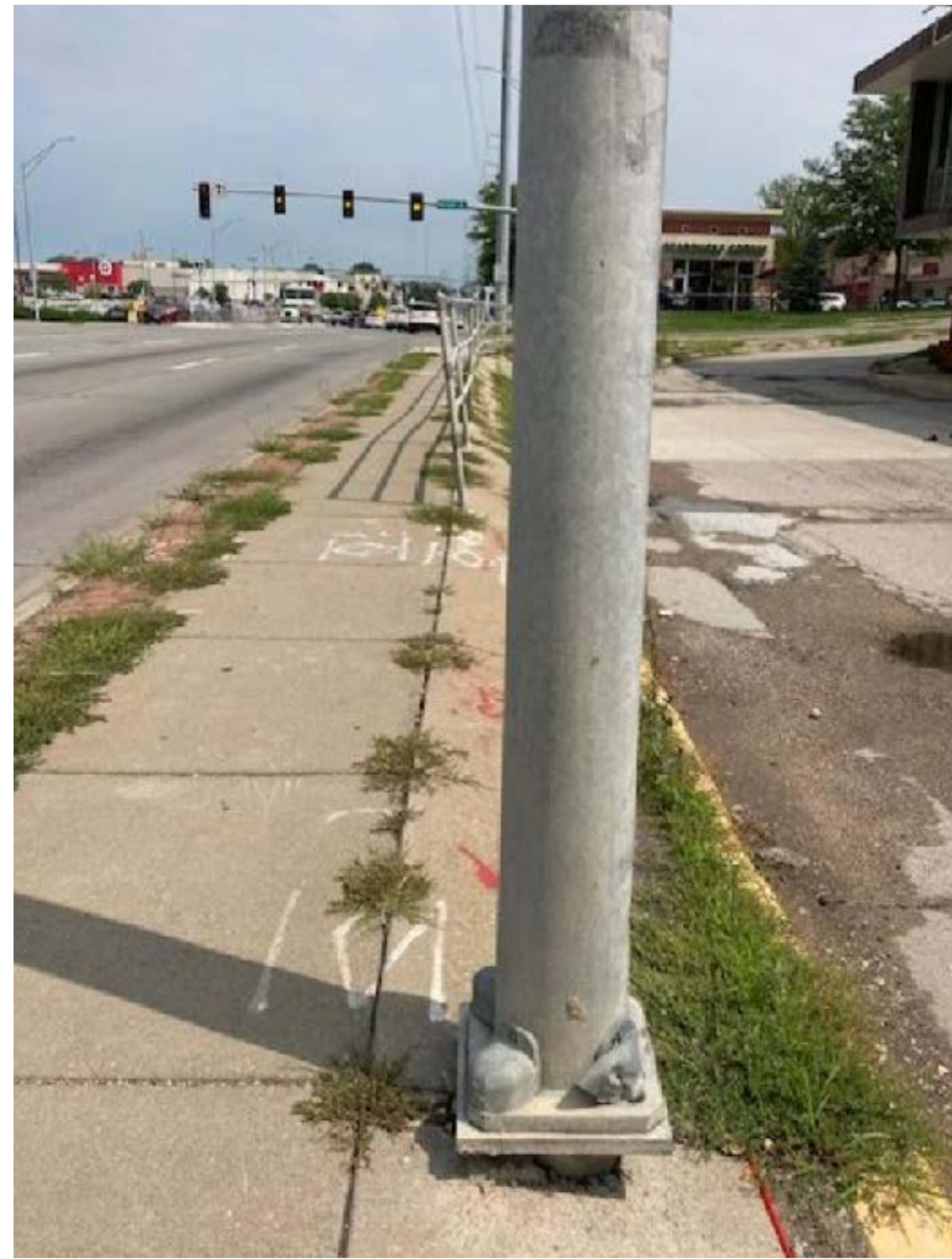
Narrow sidewalk and narrow buffer with an abundance of weeds and bent metal railing leaning into a pedestrian path.
