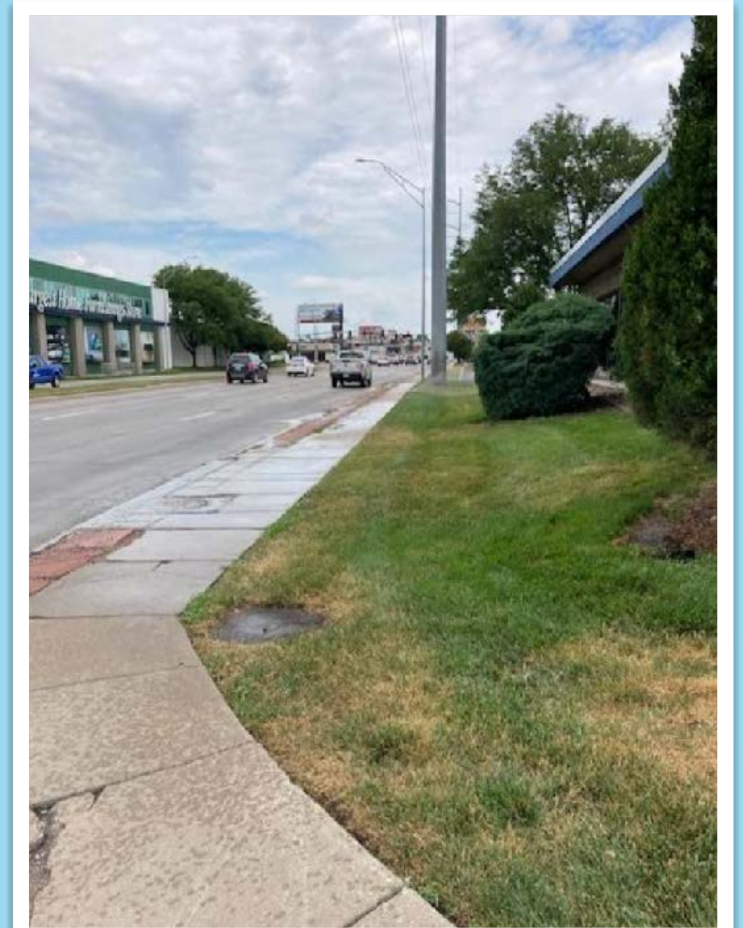
Narrow sidewalk and narrow buffer butted right up against the heavily traveled 72nd Street (east side of 72nd btwn Jones Street and Rose Blumkin Drive)
