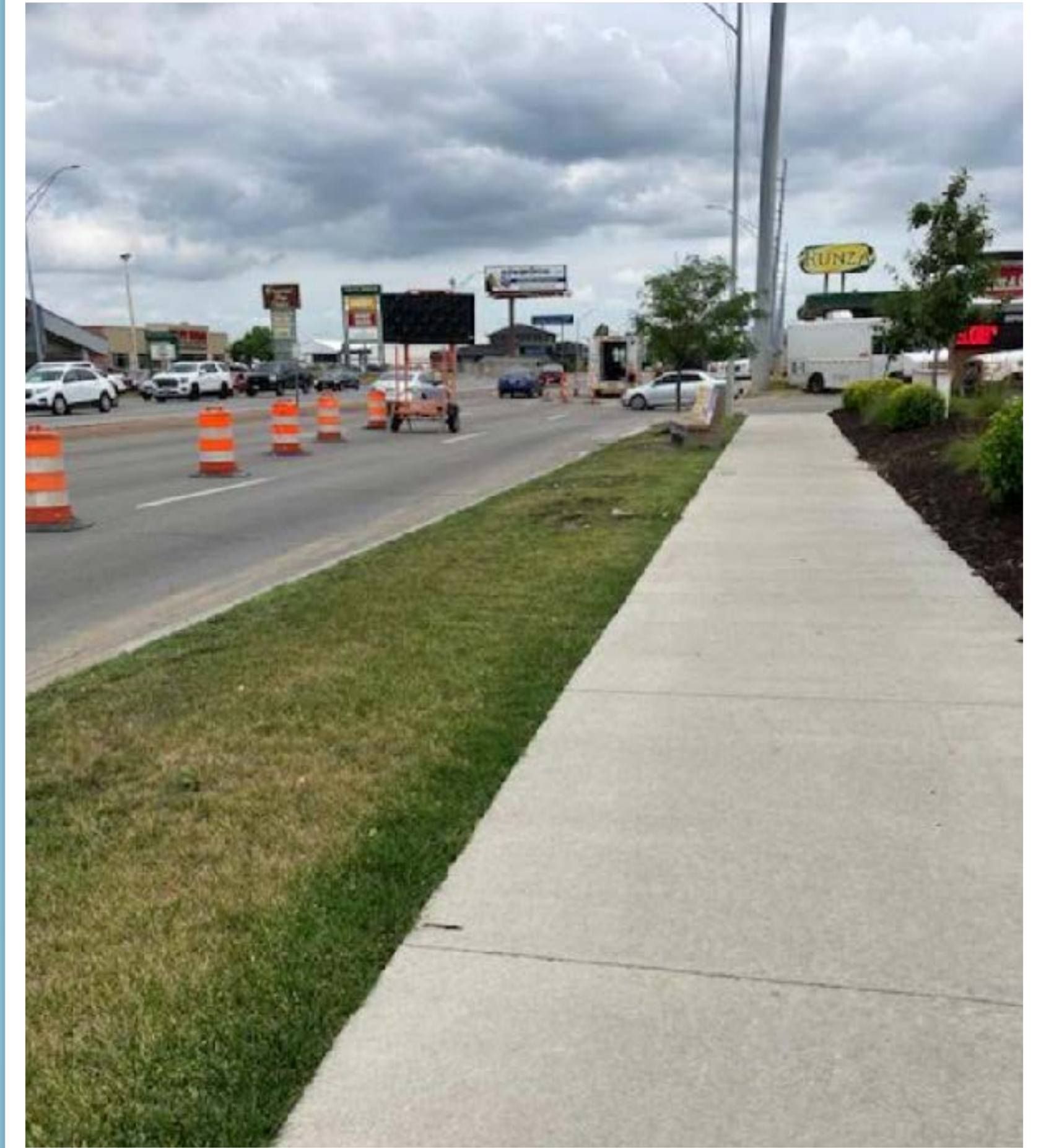
A 7-foot wide sidewalk and ample buffer made survey respondents feel safe and protected .
